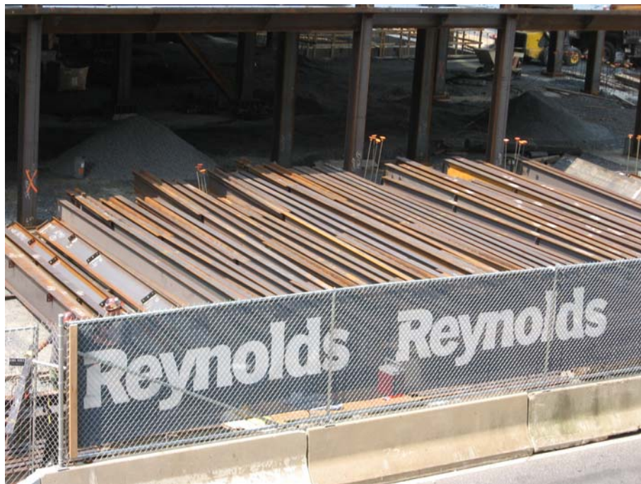
Steel Staging on Market Street
